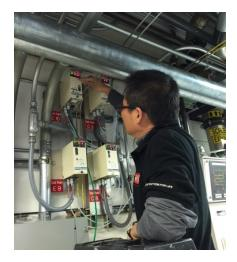
Mount transmitter in a location that can be easily accessed.
